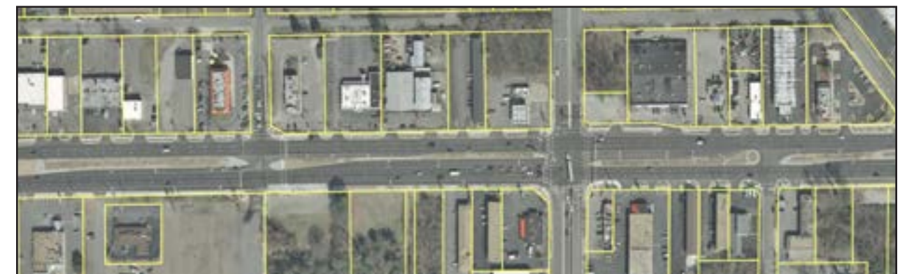
Numerous curb cuts along the north side of Midlothian Turnpike near German School Road disrupt safe pedestrian use of sidewalk.
